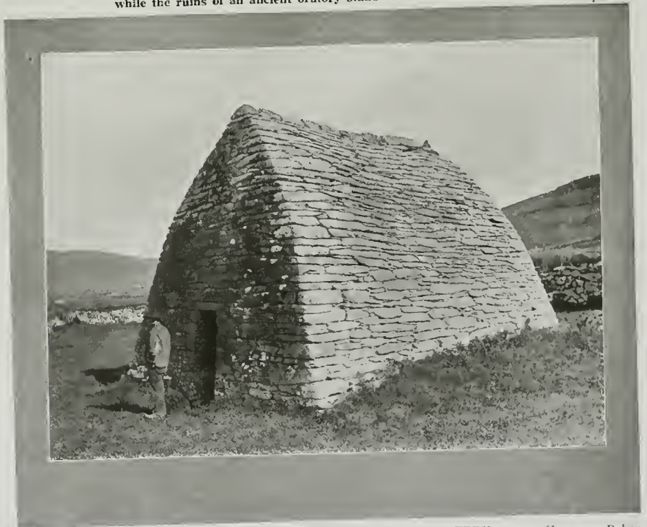
Photo by ORATORY OF ST. GALLERUS, DINGLE, CO. KERRY. [ Lawrence, Dublin. ] Situated near the romantic coast of Dingle Bay, this strange relic of antiquity dates from the seventh century, or even earlier. It is constructed of dry rubble masonry and is an excellent specimen of this crude form of architecture. Within, the faces of the stones are all cut to shape. There is an east window, above which are three pegs, probably once used for holding lamps or satchels containing hooks.
